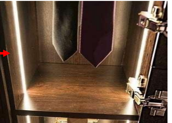
Light grooving on both the sides of verticals left and right on sensor
